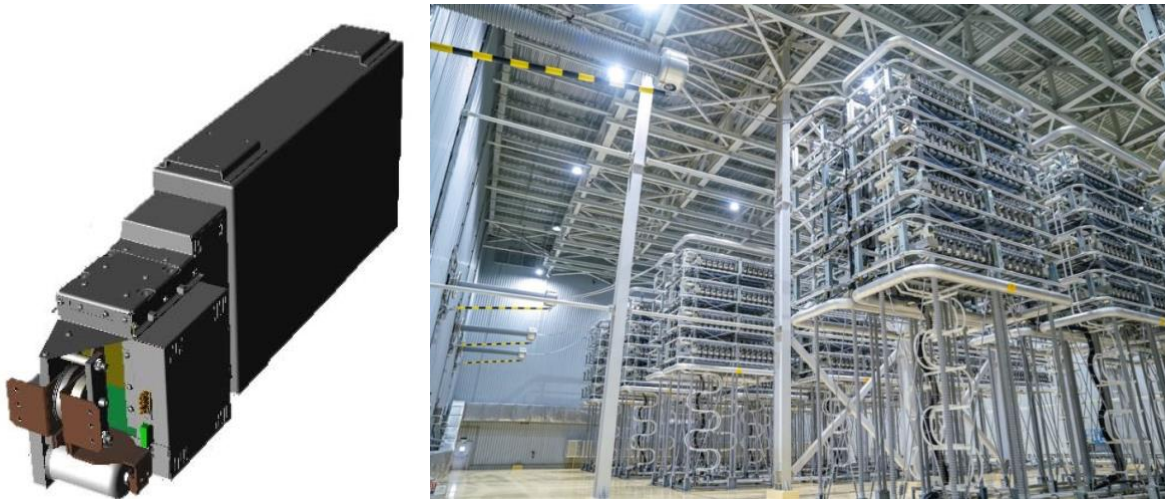
Figure 11 : HVDC submodule (left) and corresponding converter towers (right). Illustration from Siemens Energy [3].
