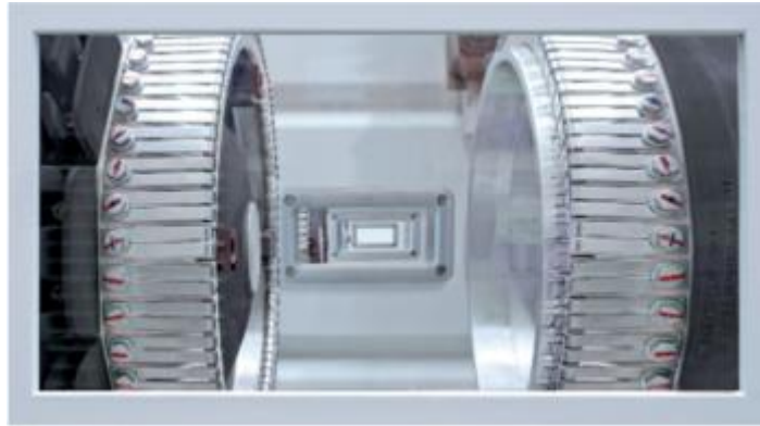
Figure 44: Example of a Generator Circuit Breaker disconnecter
